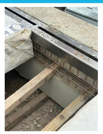
A silt collection tray is inserted in the Hydroraft before the initial Hydro block. The silt collection tray prevents, soils, sediments & metals from entering the Hydrorock drainage system.
